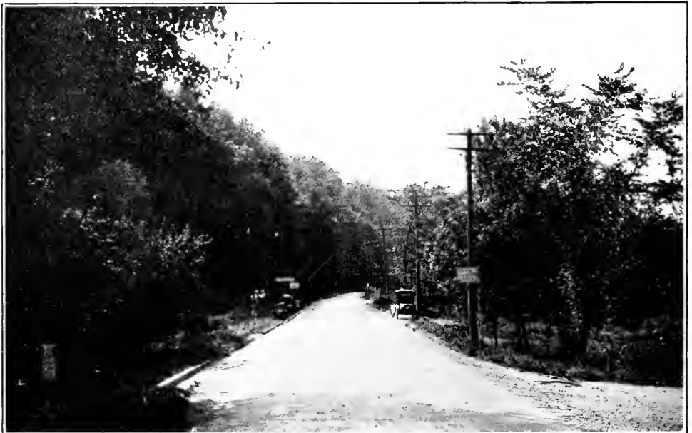
HAMILTON-QUEENSTON PROVINCIAL HIGHWAY
